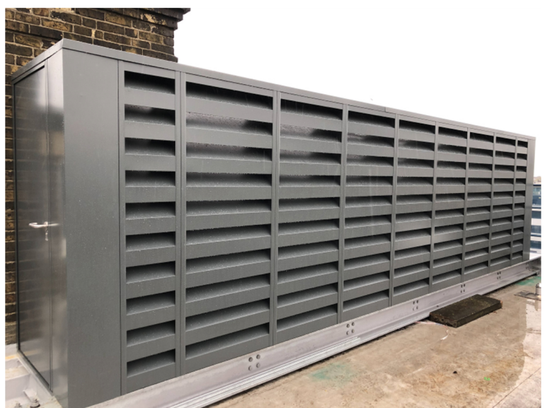
Figure 4 - Acoustic Louvre Enclosure with Single Leaf Door.
